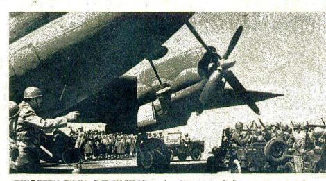
THIRTEEN FEET, SIX INCHES is the diameter of the constant speed, selective pitch, four-way feathering electric propellers used on this plane.
