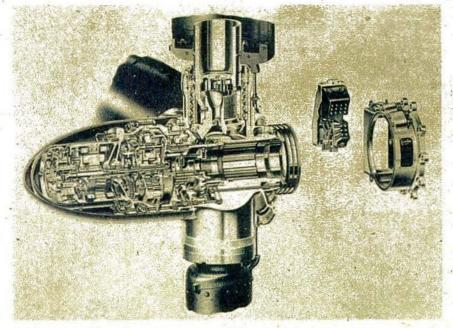
CUTAWAY VIEW showing revision mechanism of 4-way hollow steel or aluminum alloy blade propellers. Curtiss principle permits turning blades all the way around into reverse angle. Four-blade types are used on fast, high altitude fighter, bomber and cargo planes, su h as Republic P-47 Thunderbolt, Martin B-26 Marauder, and the Curtiss C-46 Commando.
